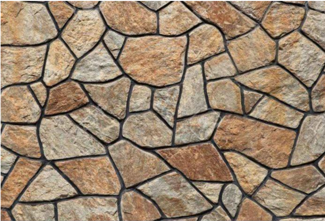
Random Rubble Stone Masonry Wall
