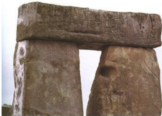
Stonehenge - trabeation detail Source: Trachtenberg & Hyman
