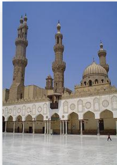
The courtyard consist of point arch with marble column and stucco ornamentation
