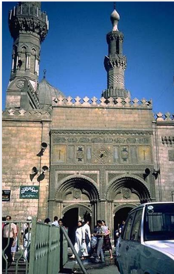
Main portal consist of double semi circle Keel arch
