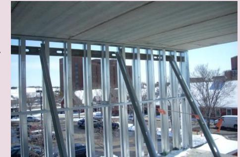
Lightweight steel studs are used to build interior walls.
