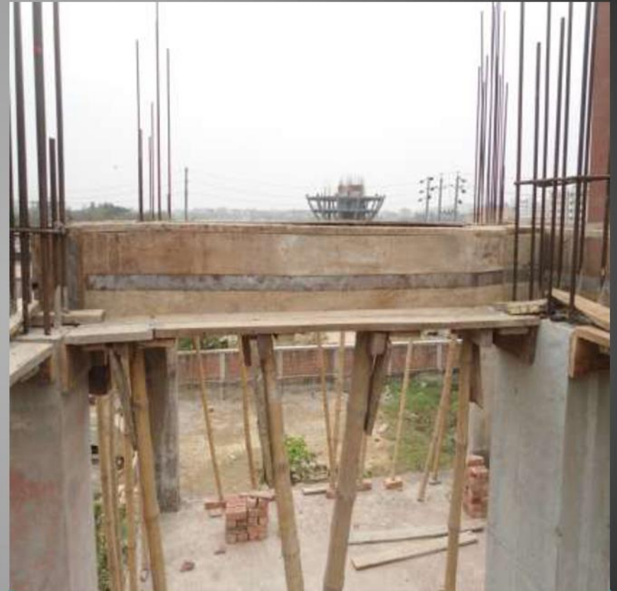
WOODEN FORMWORK
