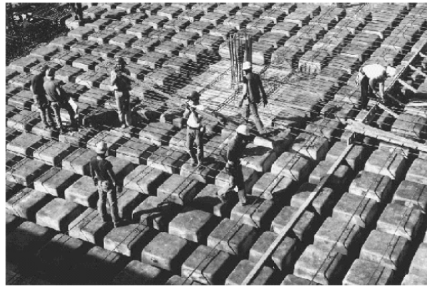
Two-way joist (ribbed) slab under construction with steel dome forms.
