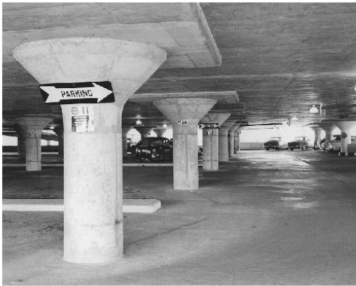
Flat slab garage floor with drop panels and column capitals.
